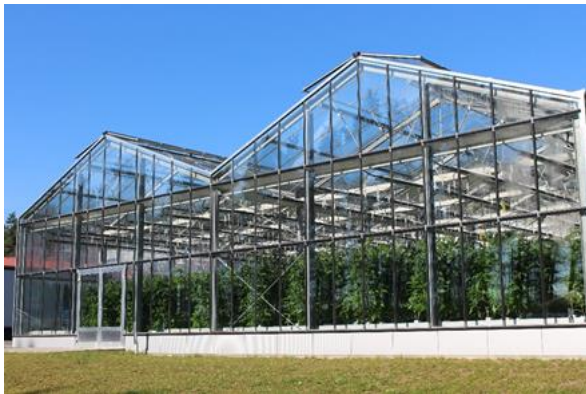
The greenhouse of the INAPRO demo-site in Waren
